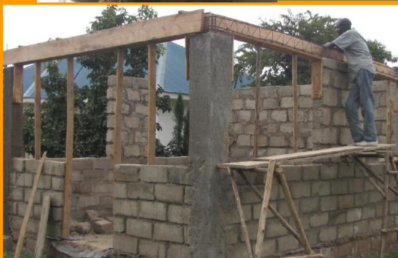
ANTENATAL AND FAMILY PLANNING WAITING SHADE UNDER CONSTRUCTION
