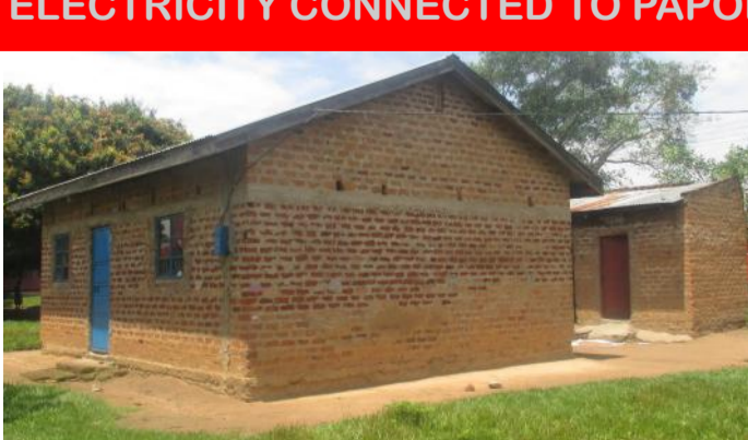
Papoli Lay reader's house
