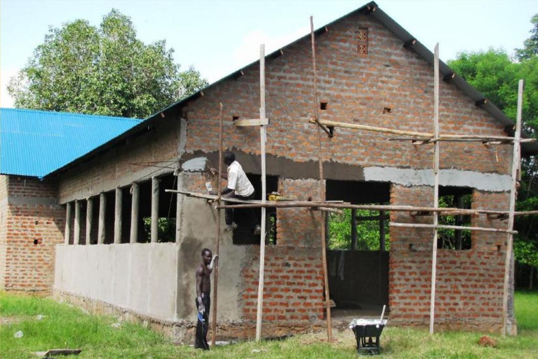
On Monday last week the plastering of the dinning hall began with most of the work centered around and inside the hall walls. According to the contractors this activity will go on for close to one week after which the wiring for electricity will be done, next will be shuttering and flooring. After which painting both inside and outside will be done and finally furnishing.
